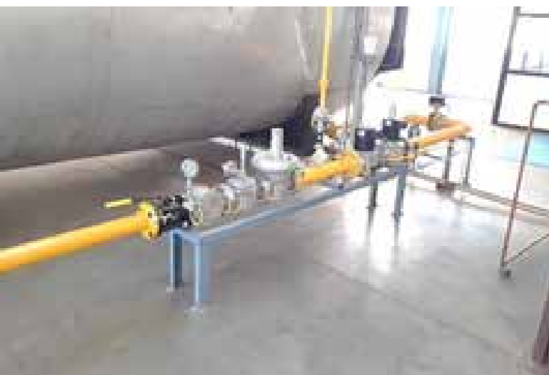
Boiler fuel conversion from HSD to PNG
